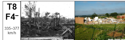
Photo: Bernd Bräuninger Ruined beech trees with distinct partial debarking. Tornado 01.06.1927 – Auen (Germany). Photo: Simon Banger Prefabricate house with brick facing blown down. Tornado 03.08.2008 – Hautmont (France).
