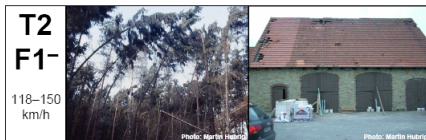
Photo: Martin Hubrig Permanently bent spruces. Downburst 06.06.1998 – Steinfurt (Germany). Photo: Martin Hubrig Roof partially untiled. Tornado 17.01.2007 – Meile-Reimsloh (Germany).
