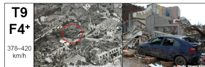
Photo: Martin Hubrig Largely debarked tree. Tornado 10.08.1925 – Borculo (Netherlands). Photo: Simon Banger Massive (brick) house ruined down to base walls. Tornado 03.08.2008 – Hautmont (France).
