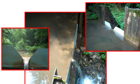
FIG. 2: View from the front, back and top of the hybrid spillway installed on the main course of Valea Băii watershed (Photo: Niță, 2009)
